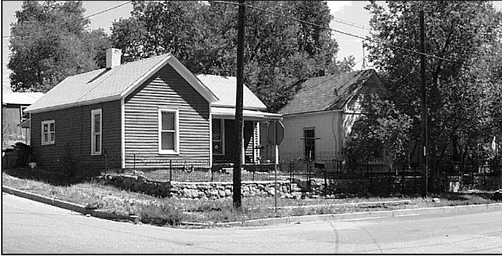
Northeast corner South Sierra Madre & Mill Street
