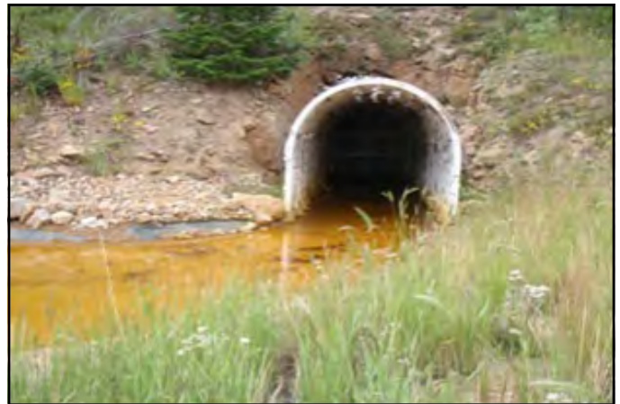
Big Five Tunnel at the Captain Jack Mill.
